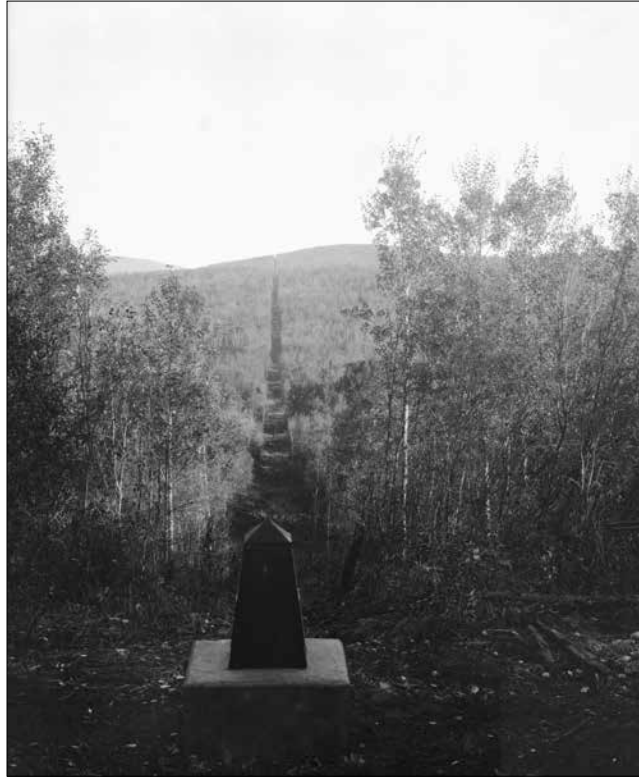
The 120th meridian line cut by Cautley's crew. e011205436, Library and Archives Canada
